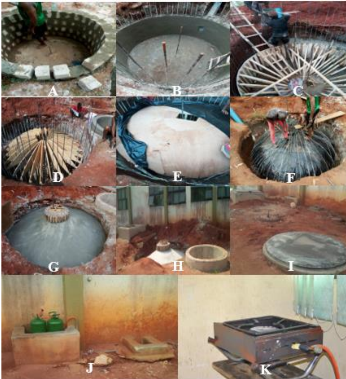
Plate 1. Construction stages of the fixed dome digester.
